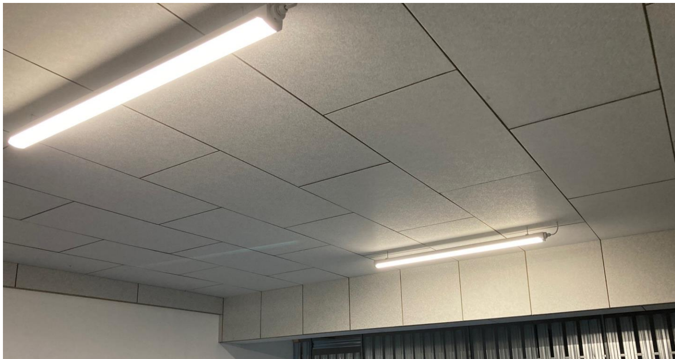
Topdec Smartline in Klebemontage
