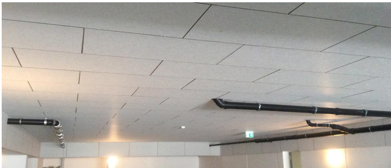
Topdec Smartline in Klebemontage
